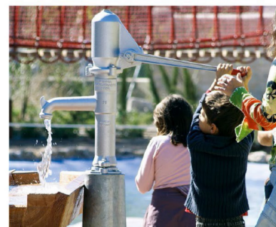
7. Pump for water play in nursery garden.
