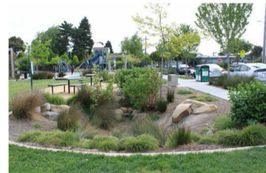
2. Rain garden retention basin
